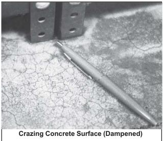
craze cracking. Avoid the delayed application of curing or even intermittent wet curing and drying after the concrete has been finished.
